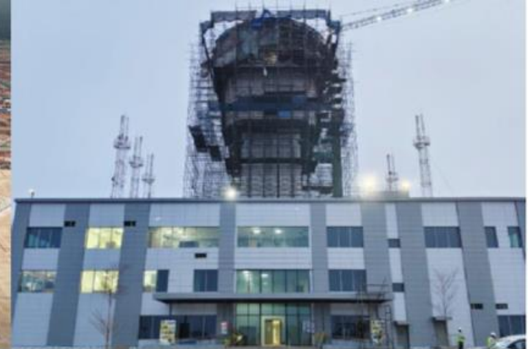
Air Traffic Control Tower
